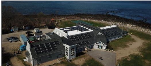
The Seacoast Science Center in Odiorne State Park received a 63.6kW solar PV system
