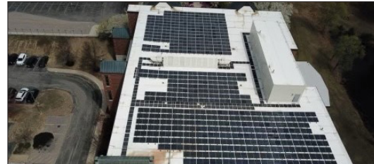
Aerial view of the Rockingham County Courthouse with roofmounted solar PV totaling 135.2 kW
