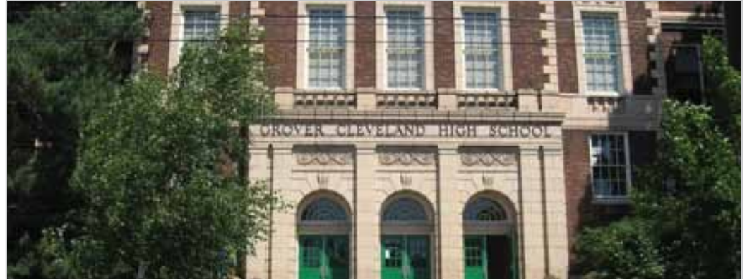
With the help of Ameresco and its proprietary process, Total System Evaluation, the Portland Public School District is updating infrastructure and reaping the benefits of cost savings with minimal capital investment through a multi-phase partnership. The Cleveland High School (above) was part of the pilot program.
