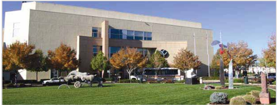
Under the energy efficiency project, Ameresco installed 12 energy conservation measures. The City benefits from improved overall energy efficiency and more reliable equipment at its facilities.
