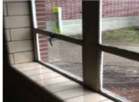
Windows at the Franklin Early Childhood Center will receive weatherization.
