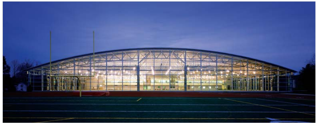
Kenyon's Athletic Center (KAC) was one of the facilities removed from the central steam distribution system, allowing for the plant to shut-down during the non-heating season.
