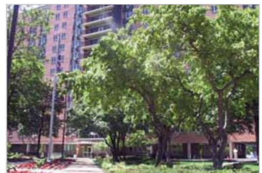
Ameresco installed HVAC upgrades under Phase 4 of the EPC with the CHA.
