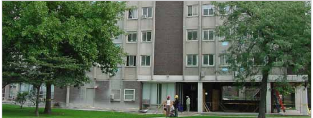
For over a decade, the Chicago Housing Authority, the nation's second largest public housing authority, has worked with Ameresco to update aging systems through energy performance contracts (EPCs) as part of the CHA's Plan for Transformation.
