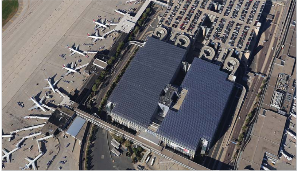
Minneapolis St. Paul International Airport 3-megawatt solar installation on the top deck of two Terminal 1 parking structures.
