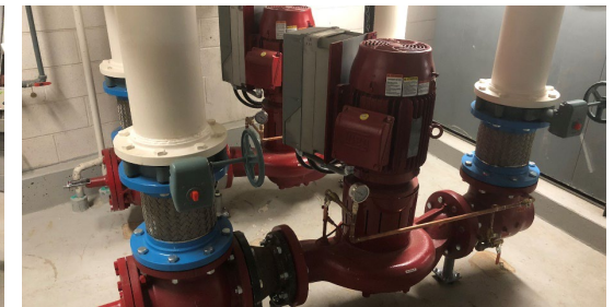
VARIABLE SPEED PUMPING
