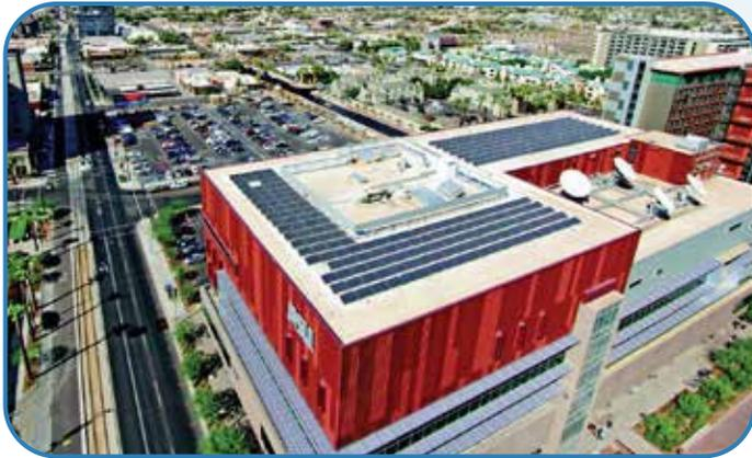
canopy arrays and ground mounted single axis tracking systems. The photovoltaic systems include 56,378 panel modules and 2,000 solar thermal evacuated tubes installed at 47 sites throughout four campuses and the Research Park. Solar canopy installations have provided over 3,904 shaded parking spaces. Ground-mounted systems cover over 18.83 acres. Approximately 29 million kilowatt hours are generated annually as a result of these
