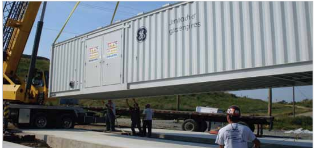
A crane sets the gas engines in place.
