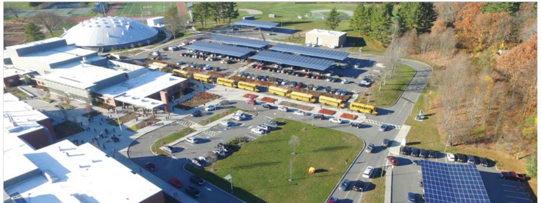
Through a Guaranteed Energy Savings Performance Contract, the Town of Wayland was able to replace old, inefficient equipment at Town and School buildings. More than 4,000 photovoltaic panels at four sites are expected to generate over 1.5 Million kWh AC of renewable electricity annually.
