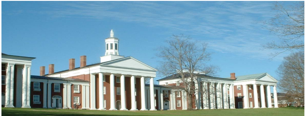
The historic university is dedicated to becoming carbon neutral and embarked on a mission to upgrade its campus to reflect this goal. Phase II of the project with Ameresco continues to be in development.
