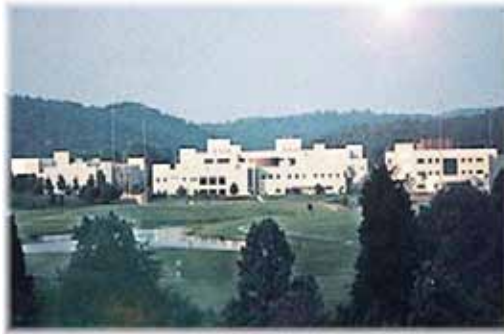
Ameresco completed work on seven member schools and is now working on two more schools for TBR.
