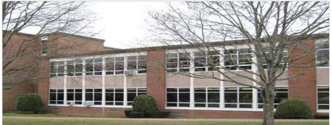
Before the partnership with Ameresco, Southeastern Regional was facing water-usage related fines and staggering operational costs.
