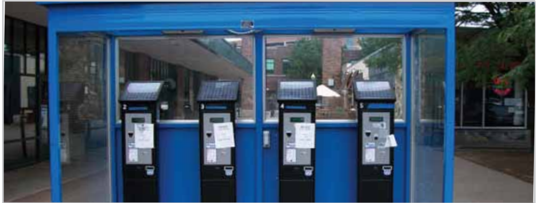
Of the 13 photovoltaic-powered parking meter shelters constructed, this was the only shelter to boast multiple meters and arrays. Above each pay meter is a photovoltaic module.
