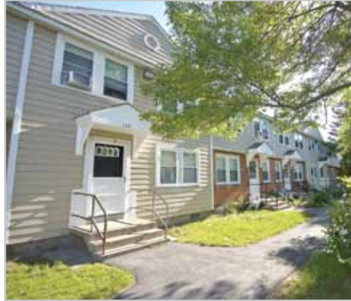
Weatherization measures will include apartment entry door weatherstripping and attic and wall insulation.
