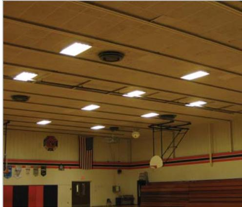
400 Watt metal halide fixtures were replaced with 54 watt T5HO high bay fixtures in the High School gymnasium.
