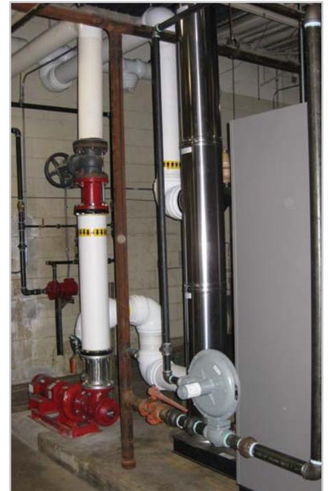
A new boiler and pumping system replaced the existing equipment, that dated back to early 1990's, at the Middle School. The new boiler also serves the adjacent Elementary School.
